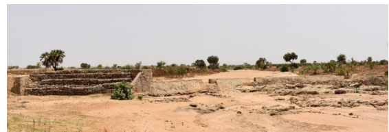
Figure 21. View from downstream of the dam
